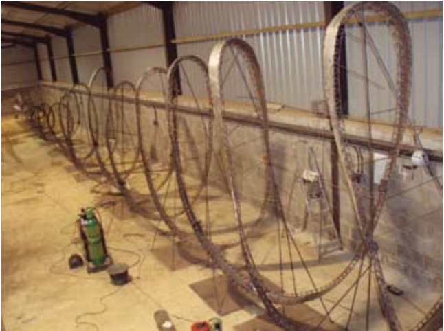
steel form for bending the wood
